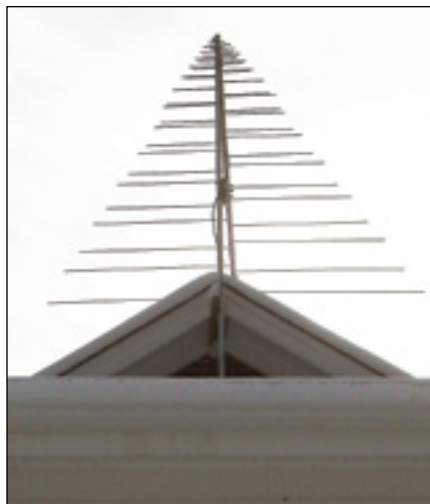
Figure 8 — The T-28 at about 35 feet looks a lot like a TV antenna while doing an effective job on six amateur bands.
